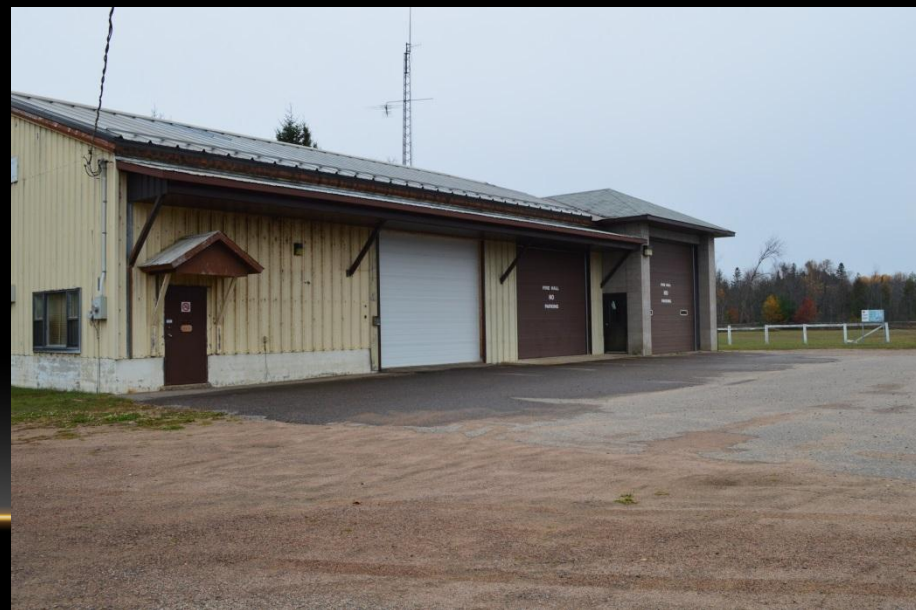
East side of Fire station
