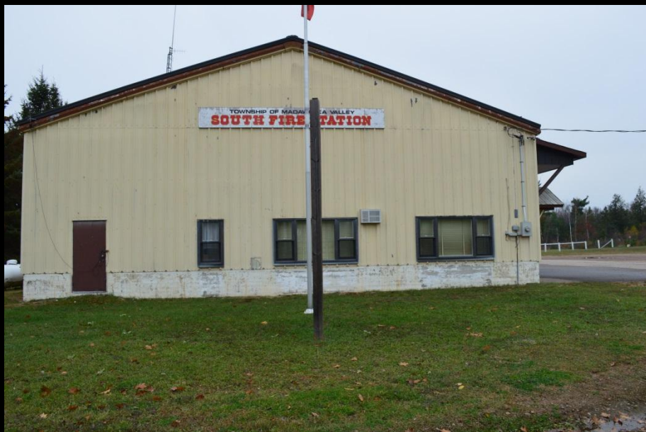
Fire station to the west of Recreation Centre
